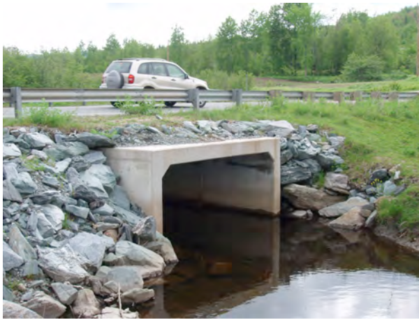
Photo 5. Box culvert at west end of Zone 9.
