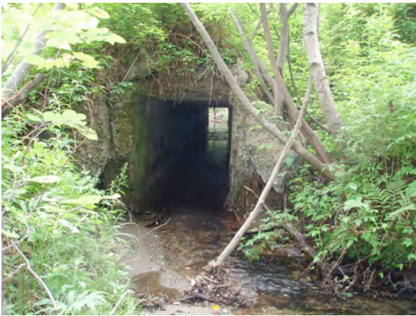
Photo 7. Existing culvert at Zone 14
