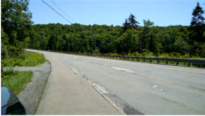
Photo 20. Line of sight from west to east
