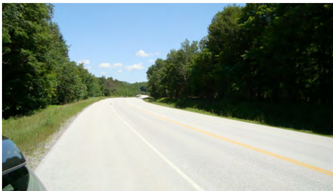
Photo 16. Line of sight from west to east
