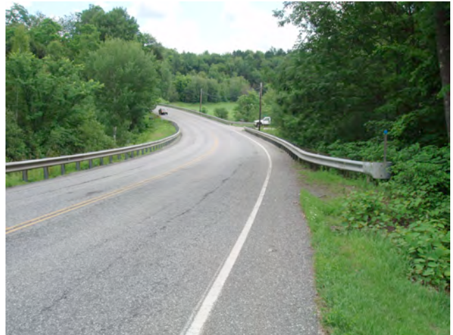
Photo 8. Route 15 above culvert
