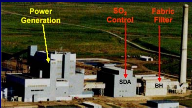
Power plant with semi-dry scrubber for sulfur dioxide control and fabric filter for particulate control.
