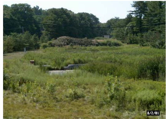
Overview of Stormwater Wetlands
