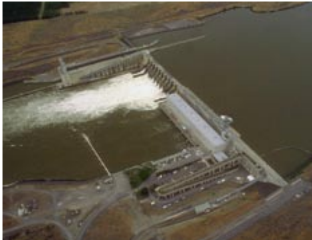
Ice Harbor Dam, Snake River, Washington. Source: U.S. Army Corps of Engineers
