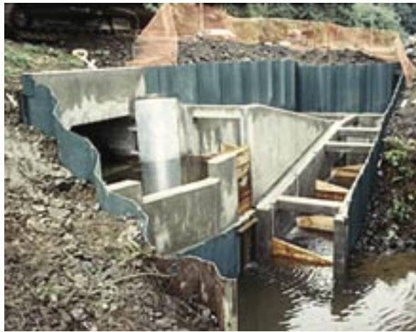
Fish ladder on a stream in Washington. Source: Washington Department of Fish and Wildlife
