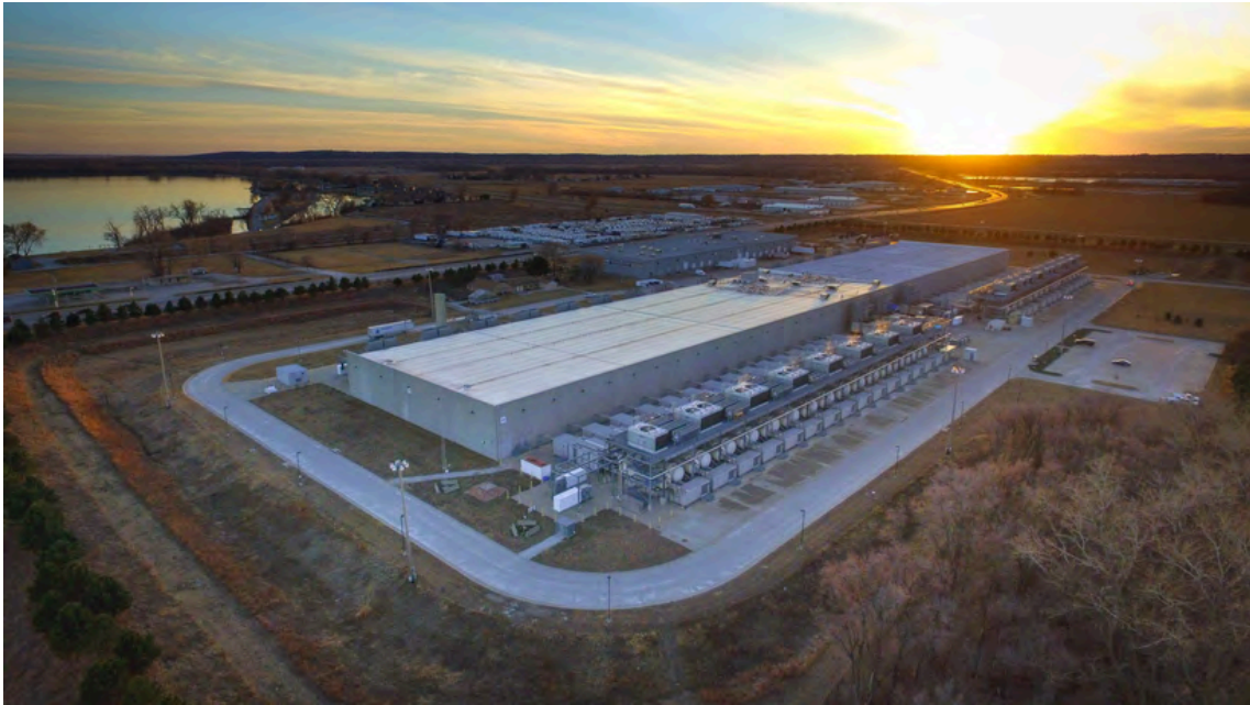
Data Center in Council Bluffs, Iowa. Credit: Chad Davis
