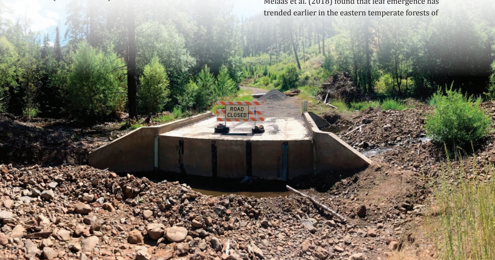
More extreme rainfall events and flooding are causing damage to roads and other infrastructure on national forests (Umatilla National Forest, Oregon). Photo: USFS.
