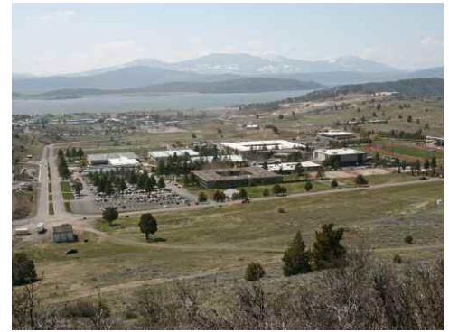
Hot groundwater pumped from wells at the Oregon Institute of Technology provides heating energy for the whole campus.
