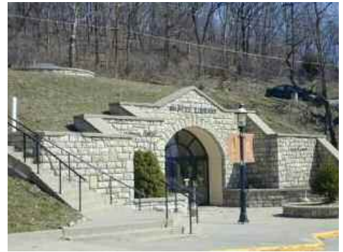
McAfee Memorial Library at Park University (MO) opened in 1988. Underground space for this building was mined into limestone bedrock.
