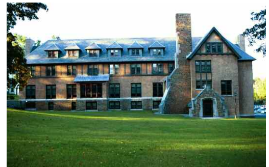
When the Skenandoa House at Hamilton College was renovated, a geothermal heat pump system contributed both to historic preservation and energy efficiency goals.
