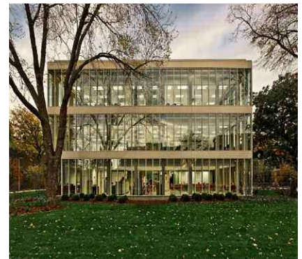
Grant Hall at the University of Illinois-Chicago installed geothermal heat pumps as part of a comprehensive energy efficiency retrofit.
