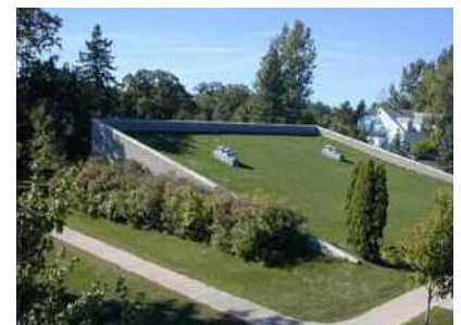
Grass-covered roof on the Seton Apartments at St. John’s.
