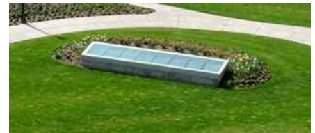
A skylight brings daylight into part of the Lokey Labs building at the University of Oregon.
