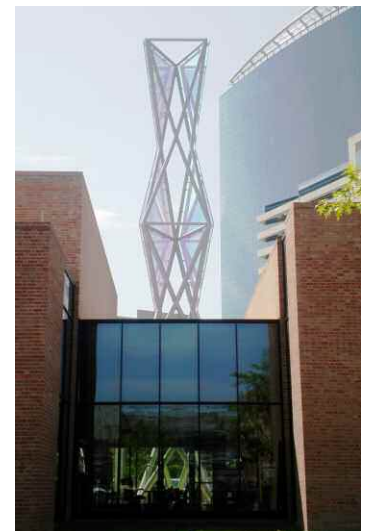
Rice University's new South Utility Plant has a small closed loop system that serves the building's glass-enclosed high-tech control room. Photo: Richard Johnson
