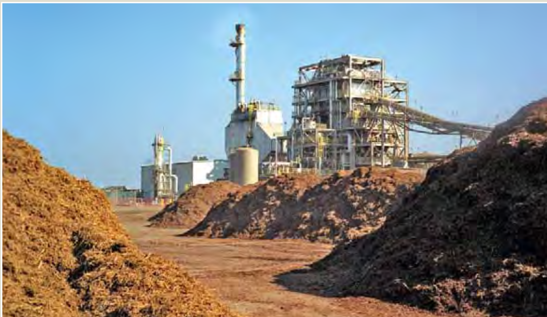
This 21 MW power plant uses fuel from wood residue
