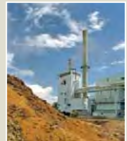
McNeil Generating Station at Burlington, VT—a biomass gasifier which operates on wood chips
