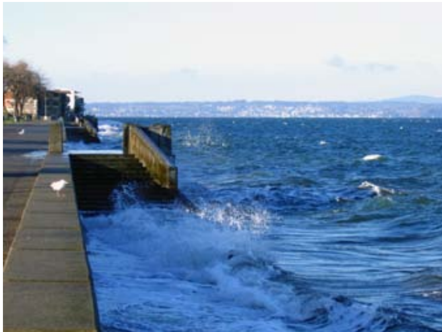
Seawall at Alki Beach in Seattle (Chas Redmond, Flickr.com)
