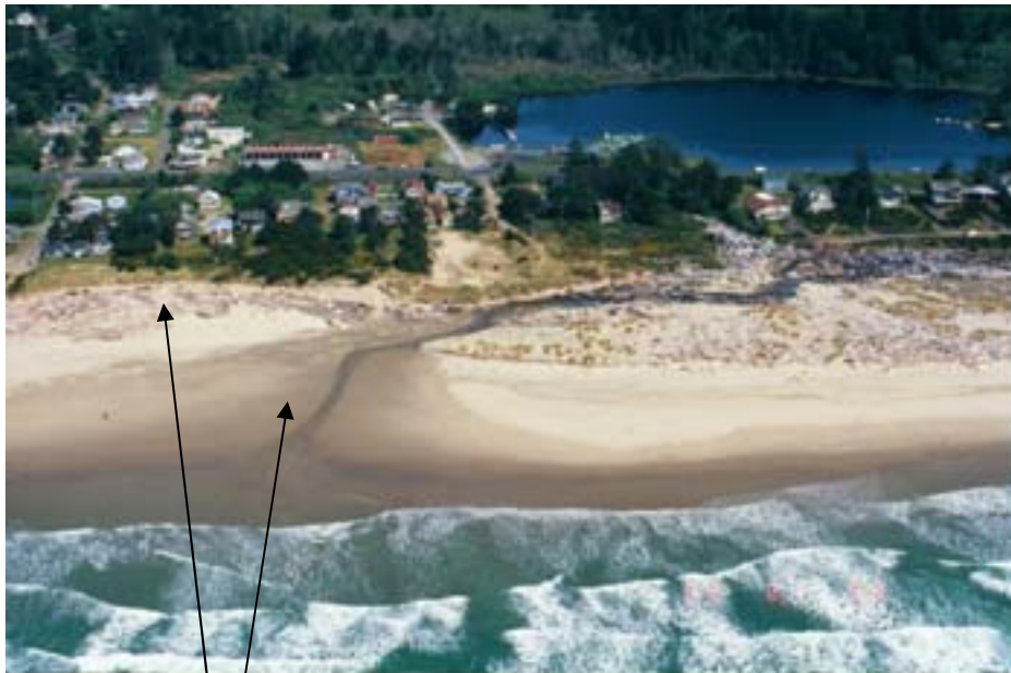
Shoreline and dune erosion
